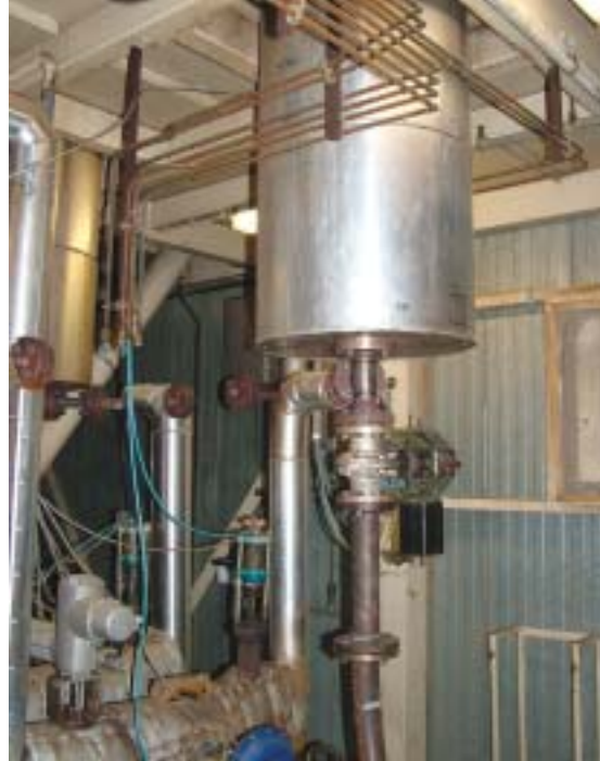
The pressure tank of the Presco system runs through a floor. Here pressure is elevated to 25 bar and temperatures rise to 300°C. At the bottom the exhaust pipe runs into the expansion tank.
