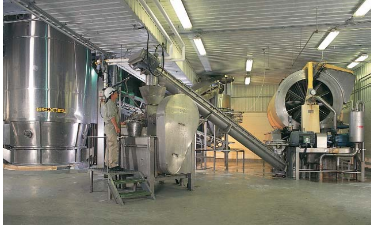
Fermentation and harvesting of fresh yeast at plant in Montreal.
